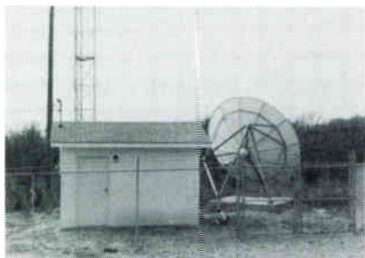
This equipment: tower, headend building, and earth station, bring hours of cable TV enjoyment to rural southeastern Missouri.
