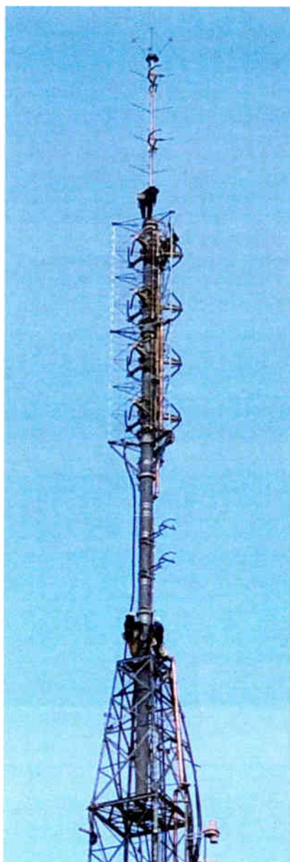
The tower with the new pole and antenna systems.
