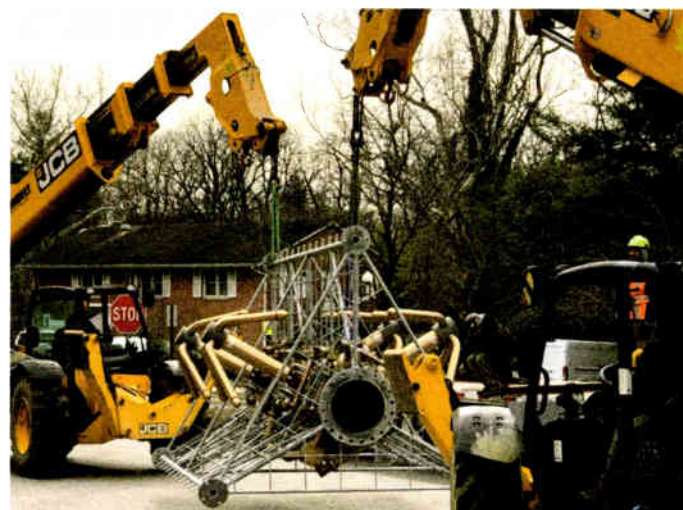
The new panel system is maneuvered through campus.
