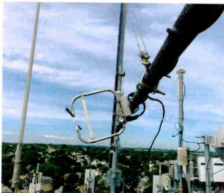
Fig. 1: The heavy-duty strut hinge joins the mast and short pipe. (Left to right: gin pole, mast mount, antenna mast.)
