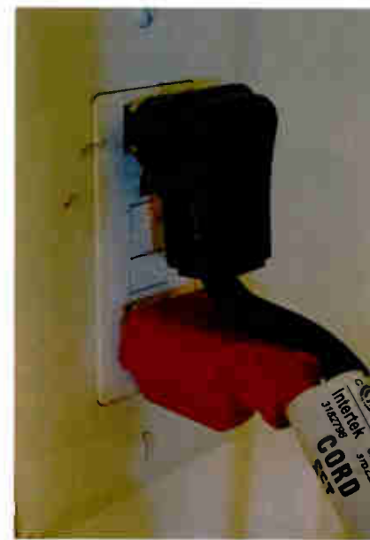
Fig. 2: Plugs may obscure the test/reset buttons.
