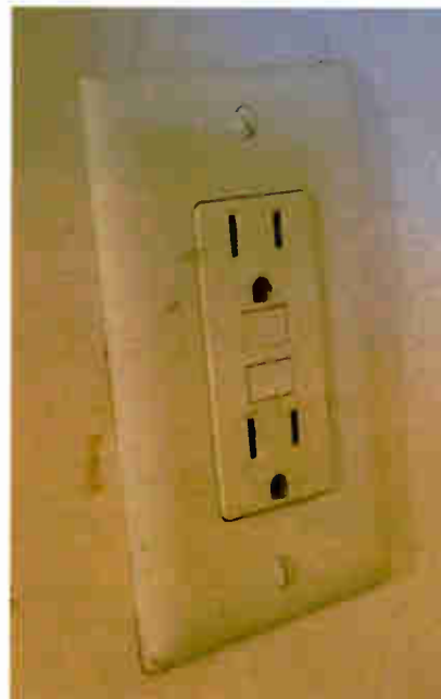
Fig. 1: The GFI "ground fault" outlet.
