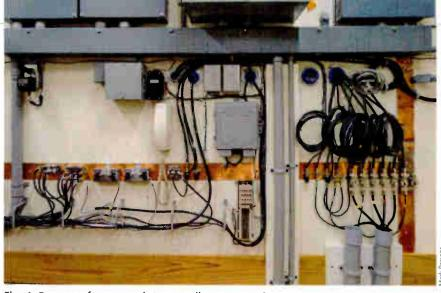
Fig. 4: Proper reference point grounding at a service entrance.
