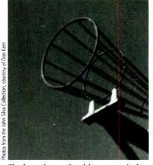
The homebrew visual (upper conical assemblies) and aural (lower split ring dipole) antennas that were used by Los Angeles TV station W6XYZ (now KTLA). It's seen on the Paramount Pictures lot but was later moved to Mt. Wilson as part of the first TV transmitter installation there.
