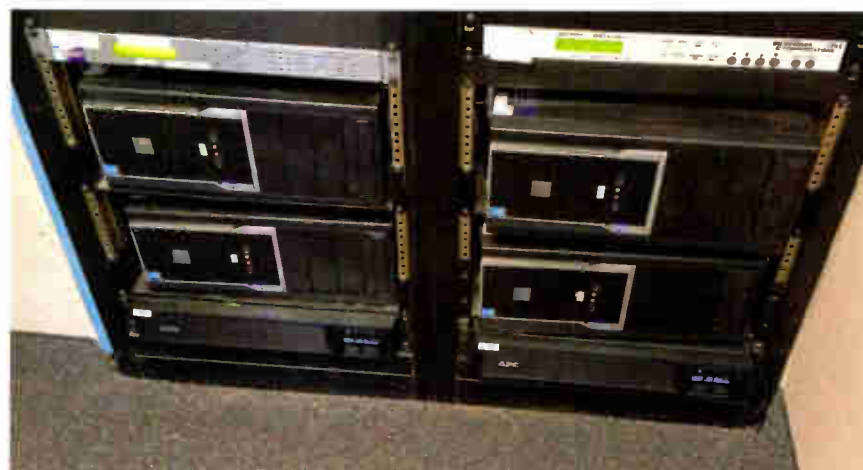
Fig. 2: Station audio output is monitored from the playout servers. (View is toward the floor.)
