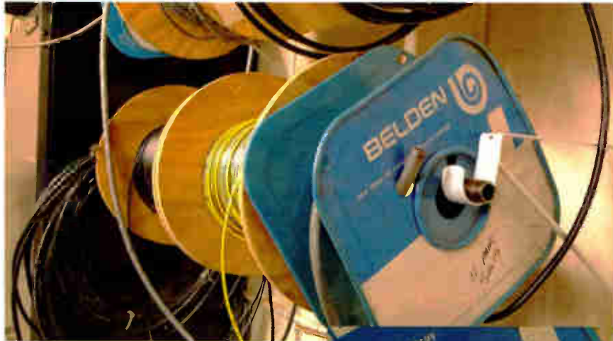
Fig. 1 (left): Wall-mount closet brackets hold reels of wire.
