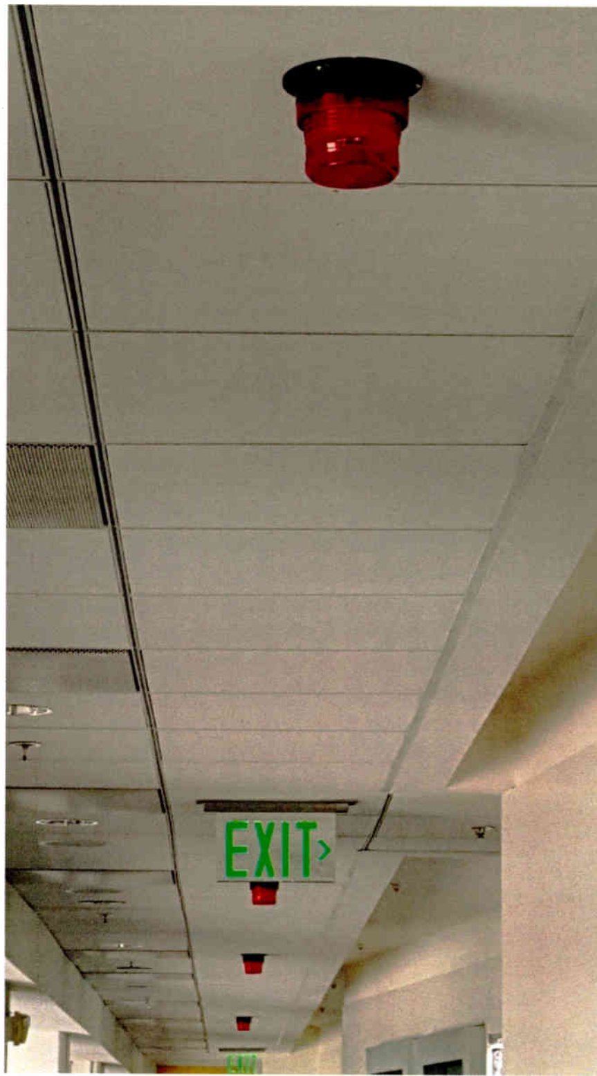
Fig. 1: Red strobe lights are tied to each studio's silence sensor.
