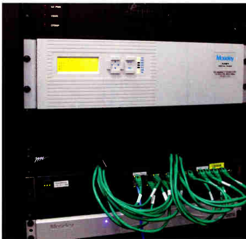
The Moseley Starlink NXE1 installed at the Oracabessa transmitter site.
