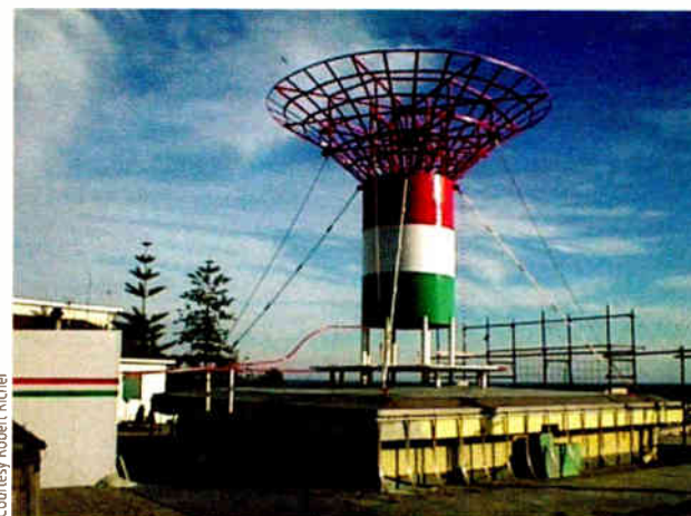
10 kW CFA installed by RAI Radio, San Remo, Italy.
