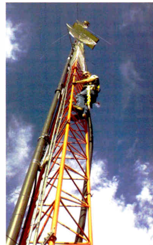
Fig. 2: Mike Payne is ready for some tower maintenance.
