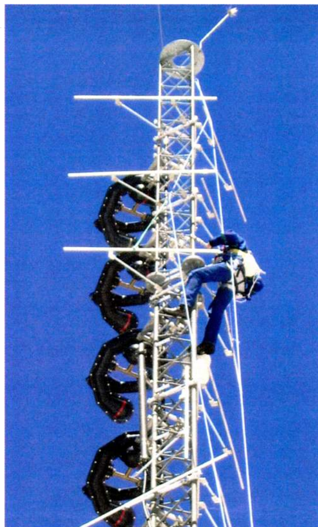
All in a day's work: Wallington en route to antenna repair.
