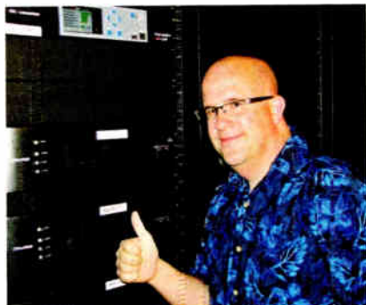
KPCC is using a Harris Intraplex Synchrocast 3 system. Chief Engineer of Southern California Public Radio Lance Harper is shown.
