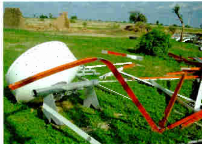
Figs. 1: The remains of this tower were scattered by high winds. In the fourth photo, we can see where bolts securing the angle iron ripped through the steel.
