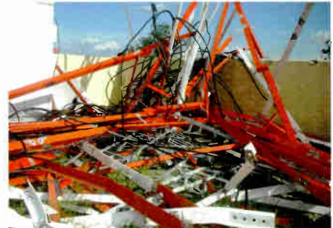
Figs. 1: The remains of this tower were scattered by high winds. In the fourth photo, we can see where bolts securing the angle iron ripped through the steel.
