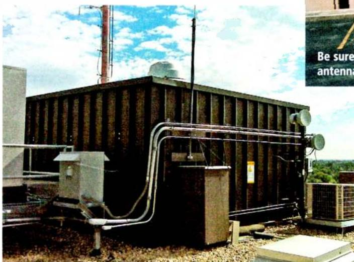
**Scout the rooftop for potential STL antenna mounting locations. Parapets and elevator penthouses often make good antenna mounts.**
