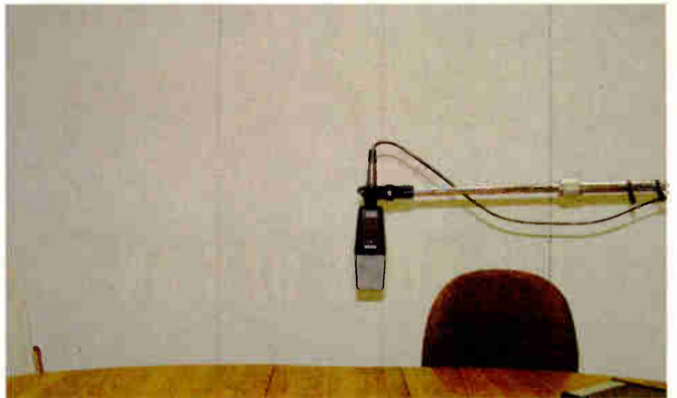
Fig. 2: Tectum is used as a wall treatment at KNLR. Routed grooves improve the aesthetics of the panels.
