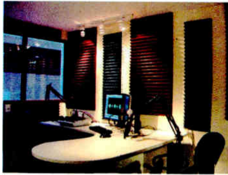
A Pleasing Installation of Absorbent Panels on a Reflective Wall
