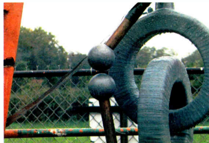
Fig. 3: The incorrectly mounted Austin Ring Transformer.
