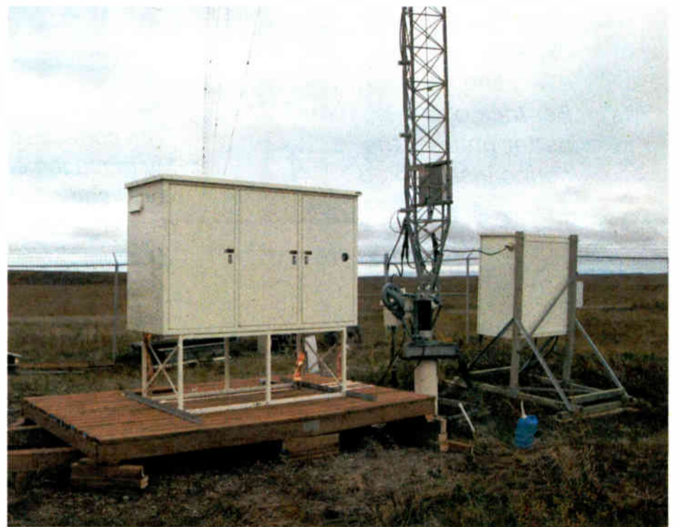
Fig. 2: A different method of mounting an ATU.
