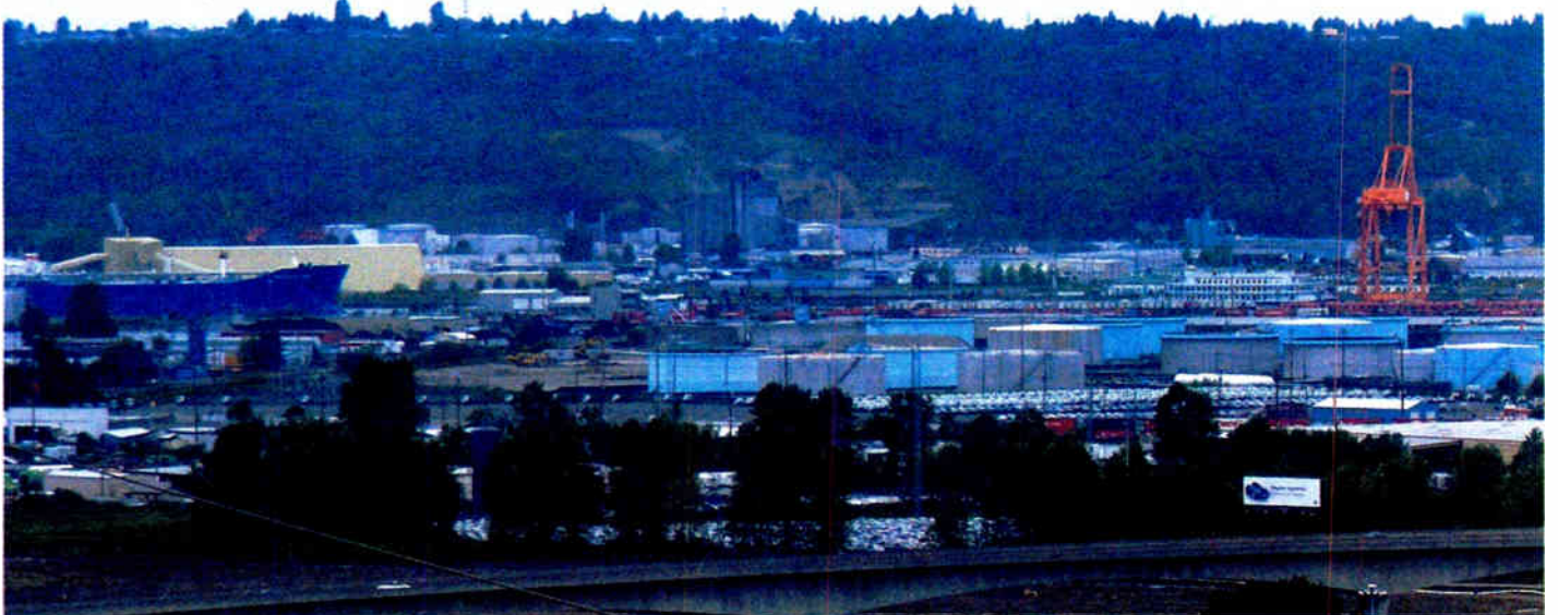
A tanker can be seen in the upper left, the refinery is center right with the tanks, and two of the KKOL towers are near the center in the middle of a car lot. The cars are new ones that have been off-loaded from cargo ships and are awaiting shipment by railcar.
