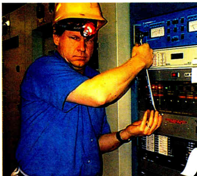
Esbjerg creates rack space to install the new ENCO server: 'I determined the directional AM controller and EAS unit being removed were probably nonessential.'
