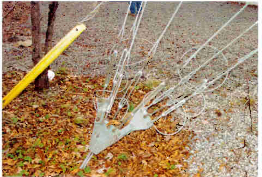
Fig. 2: Pay close attention to guy anchor turnbuckles.
