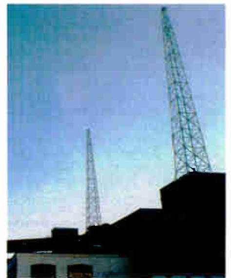
The 1921 WBZ antenna towers in East Springfield, Mass.
