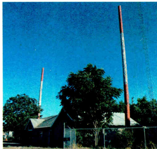
At KWG, these sawed-off poles once supported the antenna.
