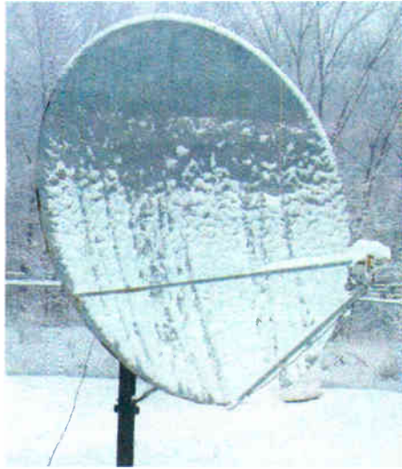
Fig. 3: A little car wax applied to satellite dishes will make even wet snow easy to remove.
