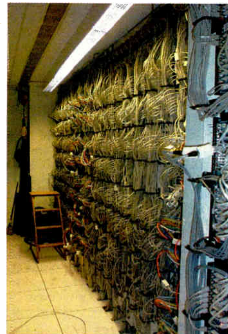
The 'back wall' IT installation of WCBS(AM) in New York includes a Radio Systems StudioHub for many of the digital audio interconnects.
