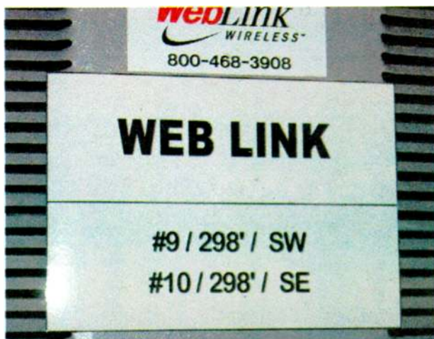
Fig. 1: Post a sign identifying lines and antennas on the transmitter.
