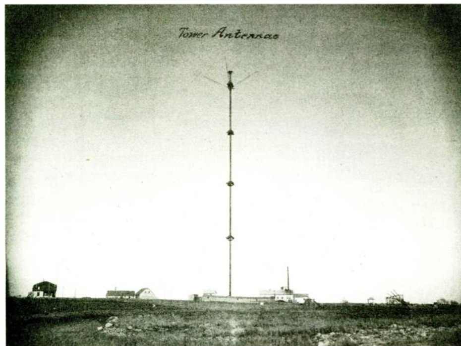
Fessenden had two identical 420-foot towers constructed at his stations in Massachusetts and Scotland. These were probably the first base-insulated guyed vertical radiators. Note the use of insulators to break the guy lines into non-resonant lengths and also the 'umbrella' top loading employed.
