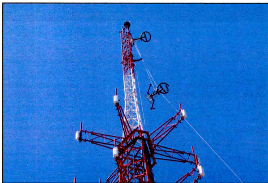
A bay of the antenna is lifted into place.
