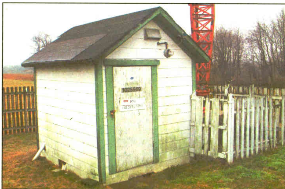
This unassuming hut is armed with a combination shock and contact unit by Ademco.
