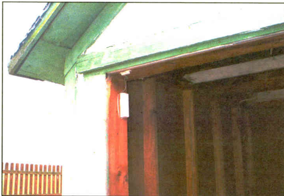
The unit uses wireless transmission in the 350 or 900 MHz range to detect the hut door opening or vibration if vandal activity.
