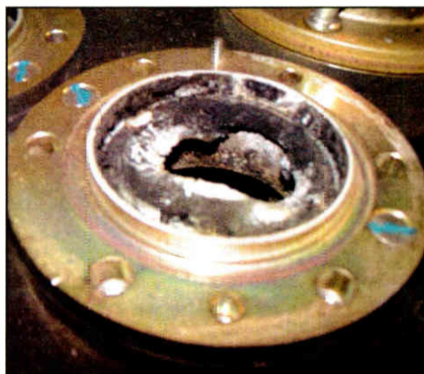
Fig. 3: Operating a transfer switch while under full transmitter power is not a forgiving event.
