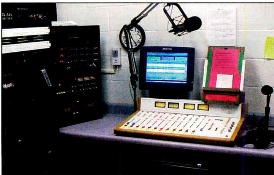
To the right of the clock is the studio's Audioarts board and Electro-Voice main mic. The racks on the left house Denon CD players, a Tascam PA-20MKII amp and a Rolls tuner.
