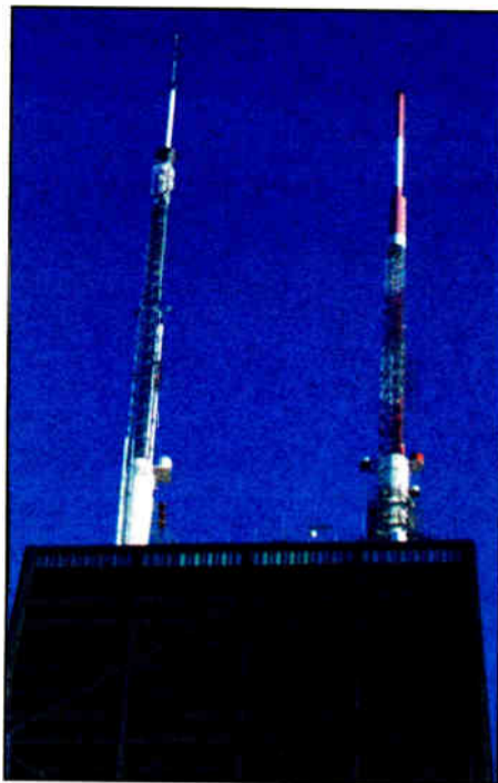
The master antenna is visible two-thirds of the way up the left tower.
