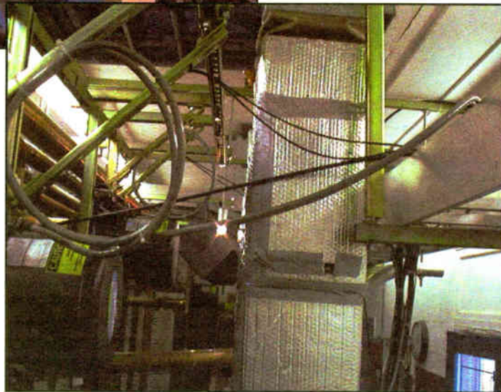
Fig. 2: Transmitter No. 2, after wrapping the exhaust stack.
