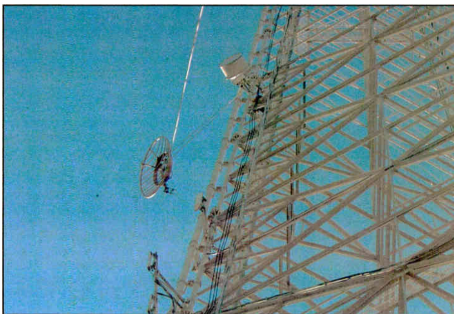
Fig. 2: The replacement dish is hoisted into place.
