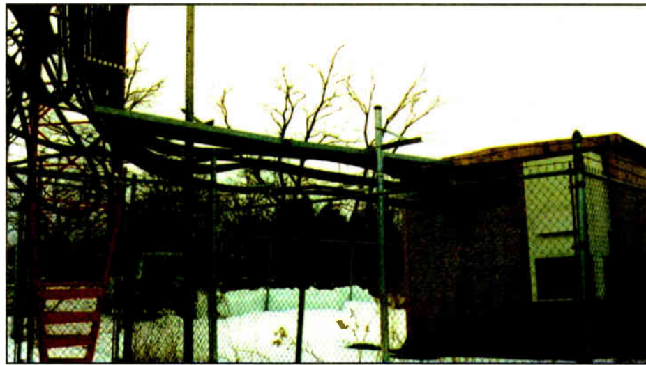
Proper T/L installation is key to reliable long-term operation.
