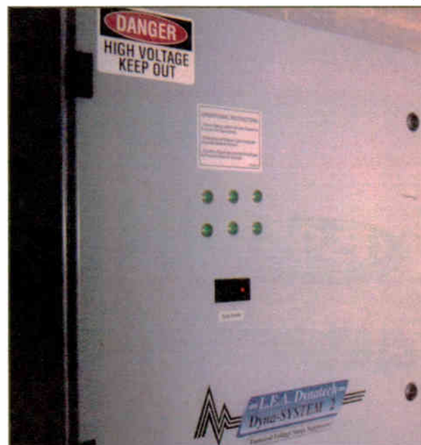
Fig. 2: Green indicators show the status protection modules on your surge suppressor.
