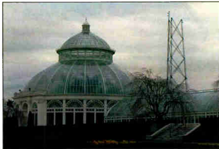
WFUV's partly constructed tower is seen from the Botanical Garden.
