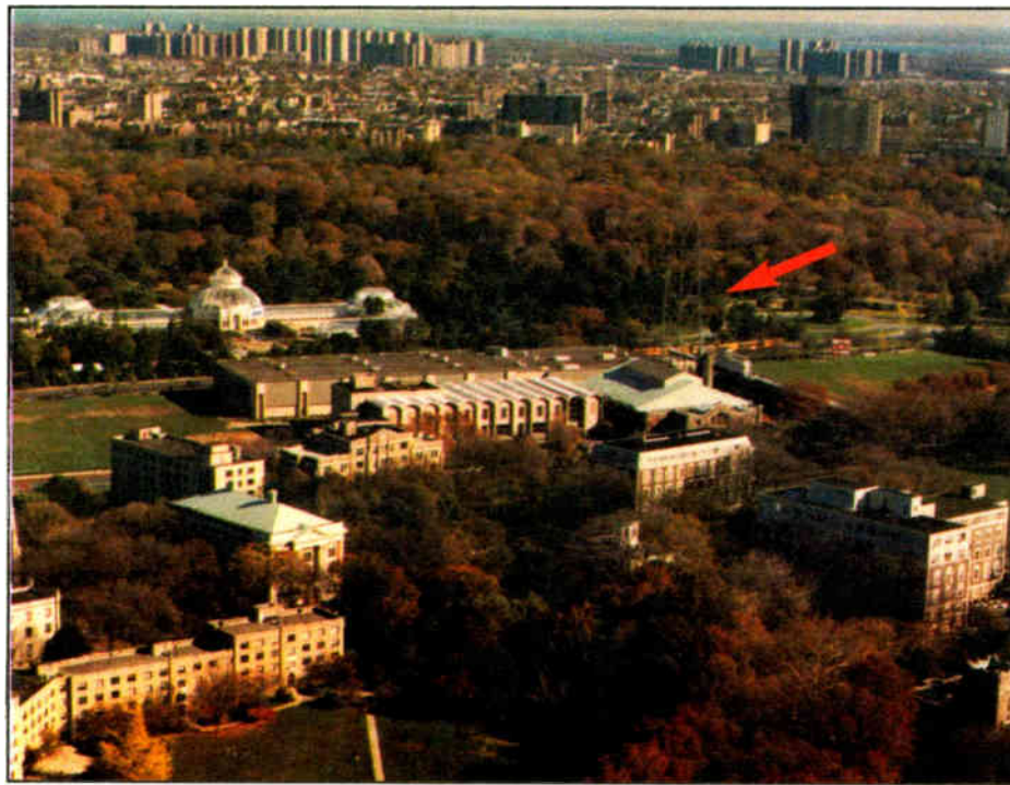
Fordham University Campus. The tower is indicated by the red arrow.
