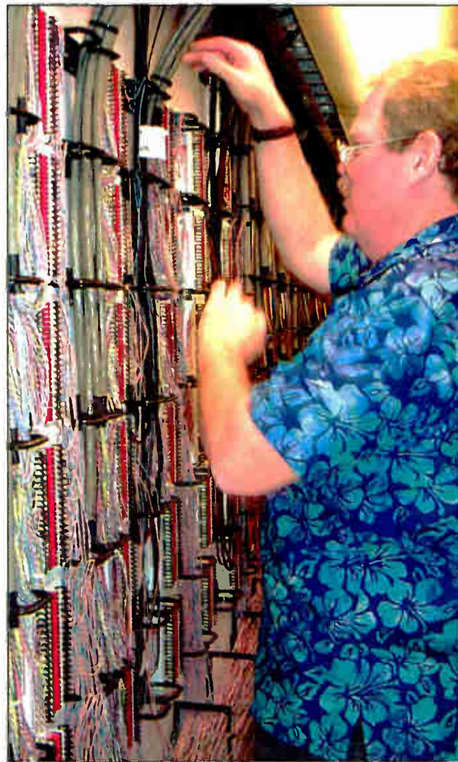
Kevin Douglass works near the main audio cable terminal wall.
