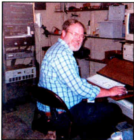
Michael Barnes is chief engineer of KVMV(FM) in McAllen, Texas. His Sage Endec EAS unit is in the rack to the left.
