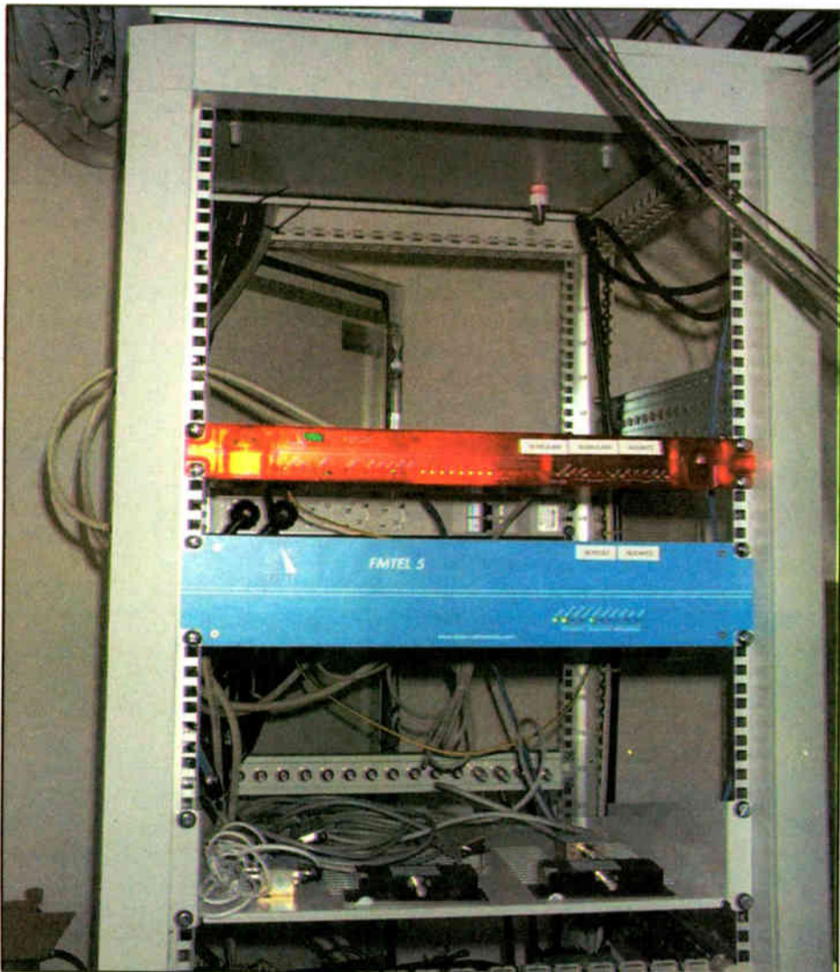
The Aztec FMTEL5-IP2port-rack is shown being installed.
