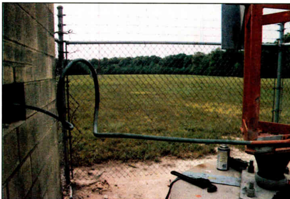
Fig. 2: A Choke on an AM Tower
