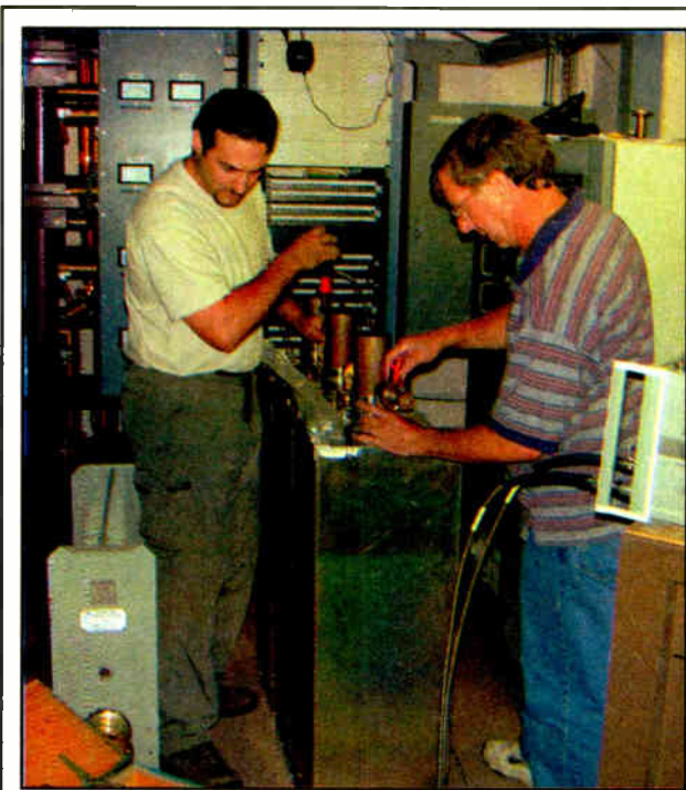
From Left: Shively's Sean Edwards and Bob Surette adjust the filter for WPAT atop the Empire State Building. After getting a call on Thursday, Sept. 13, Shively found a filter, had it tuned and on a truck by noon Friday. But the transmitter would not operate into the filter Saturday evening. Shively found the filter had changed tuning during the trek to the 85th floor. Edwards soon had the filter on frequency, allowing WPAT to operate into the broadband port of the master antenna combiner.
