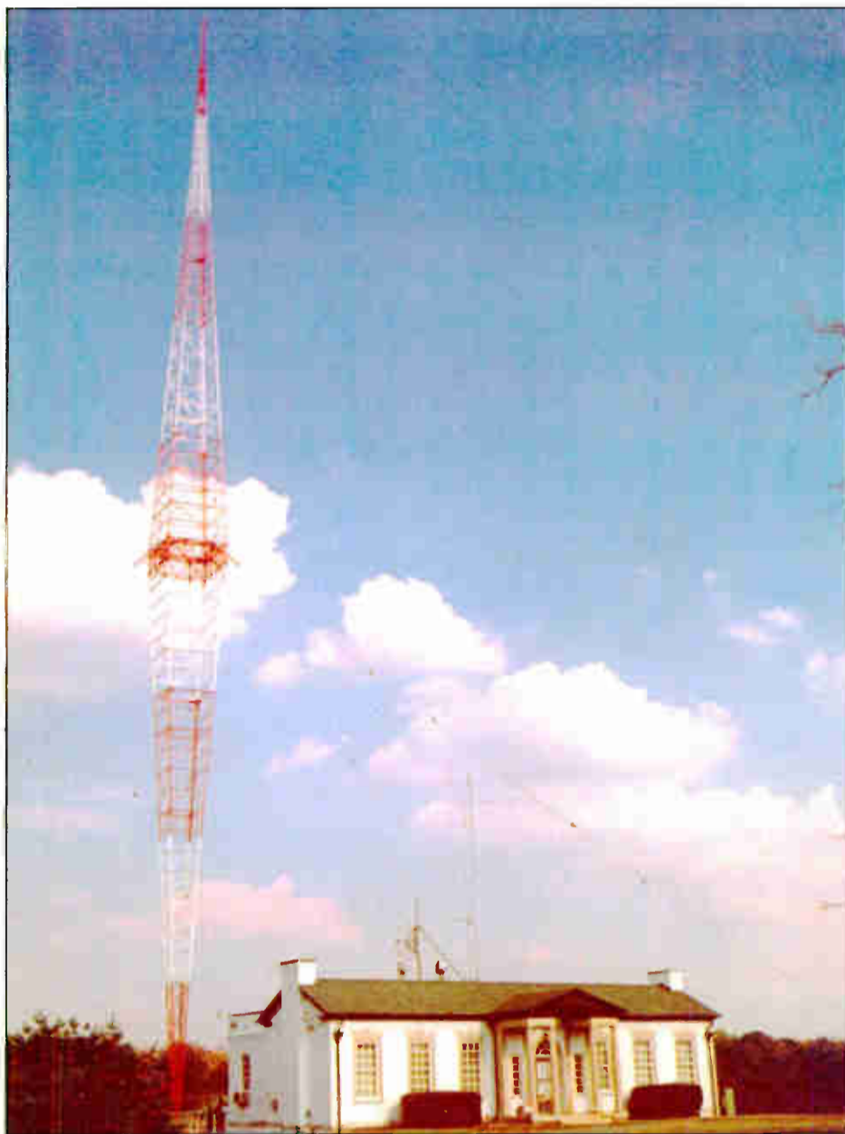
WSM(AM) Antenna Site
