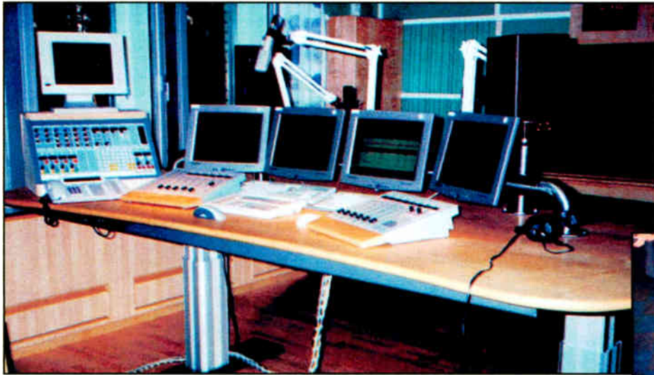
The Alice Studio. The journalist area (right) features a repositionable Seector console.
