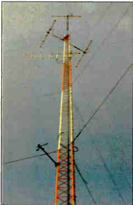
This is a view up the 125-foot tower of the interim four-antenna array. Also visible, and lower on the tower, is an anemometer (wind meter) and a back-up yagi.
