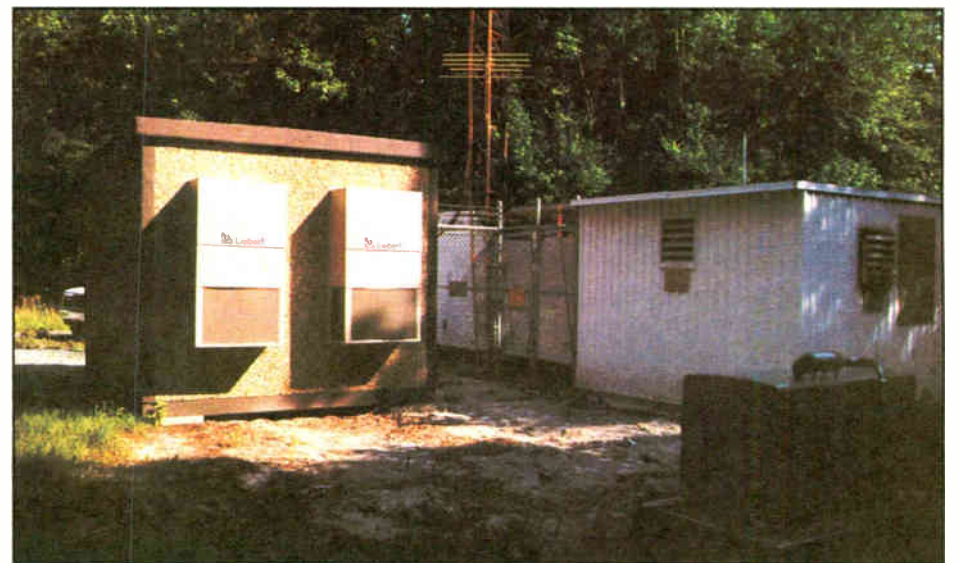
Fig. 2: Prefab buildings offer improved cooling, security and weather-tight seals
