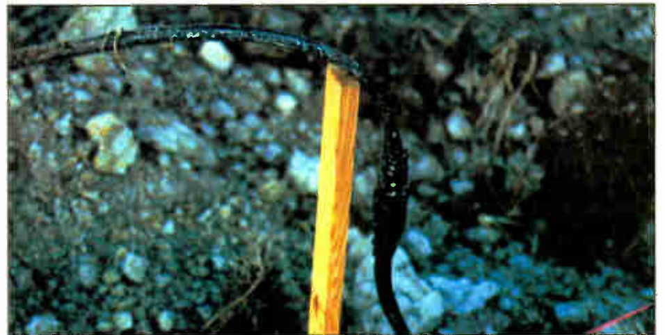
Fig. 3: Splice satellite cables properly. An electrical tape connection will permit water to spoil the splice eventually.
