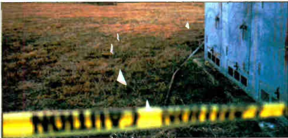
Fig. 2: Document flags or painted underground cables as provided by Miss Utility
