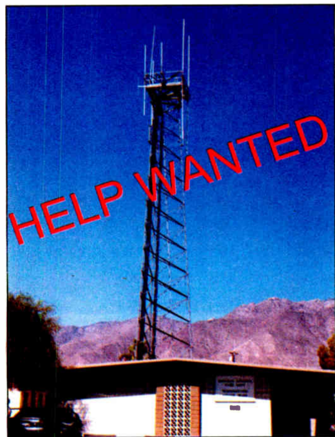
Shown is the tower site for Verizon and GTE Cellular in Borrego Springs, Calif. The building is the Borrego Springs Fire Department, which owns the tower. Broadcast must fight cellular and other industries for engineering talent.
