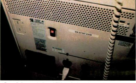
Figure 3: Keep track of new UPS batteries by noting the date on the case.
