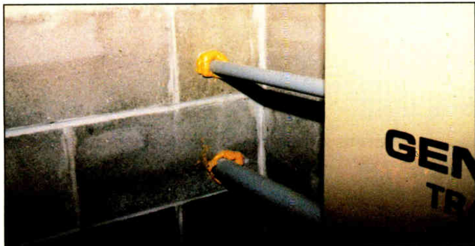
Figure 1: Sealing Transmitter Building Entry Holes
