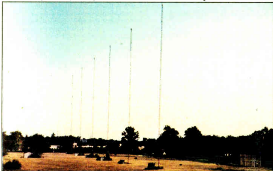
Figure 1: This AM site has vines growing up several towers, presenting a maintenance and performance hazard. A saw and a set of shears would solve this problem.
