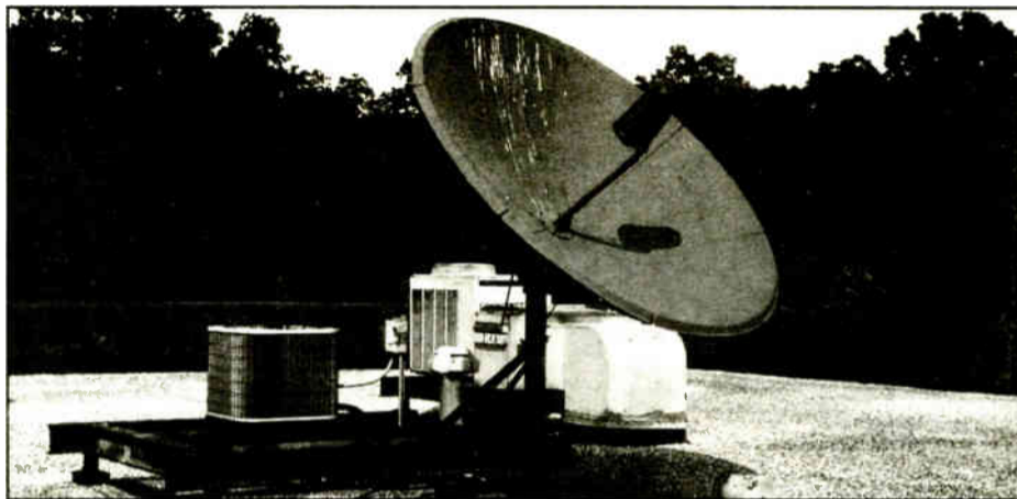
Figure 2: Keep satellite receiver dishes clean and free of pests. This one needs a wash and a coat of auto wax to prep it for winter.
