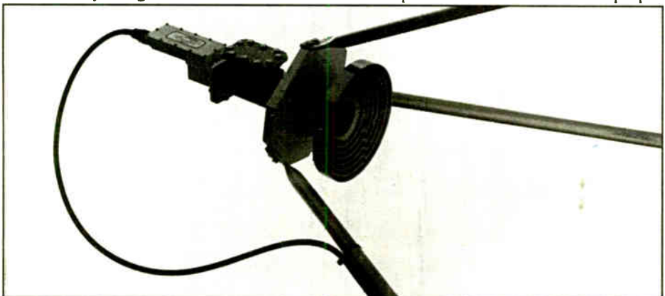
Figure 3: Check mounting bolts, cable waterproofing and the feed horn assembly before winter.
