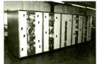
5-TOWER 50KW-U DA-2 DIRECTIONAL ANTENNA SYSTEM FOR KXTA LOS ANGELES, CA
