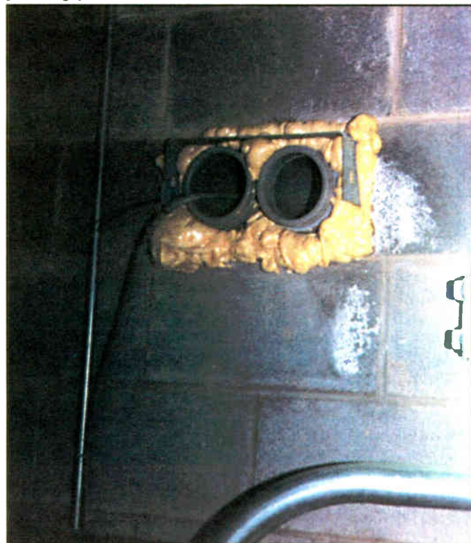
Figure 1: Seal a site to save time and money in repelling rodents and insects.
