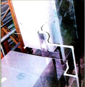
Figure 2: The extra expense of a condensate drip pan can save thousands of dollars should the drain clog.
