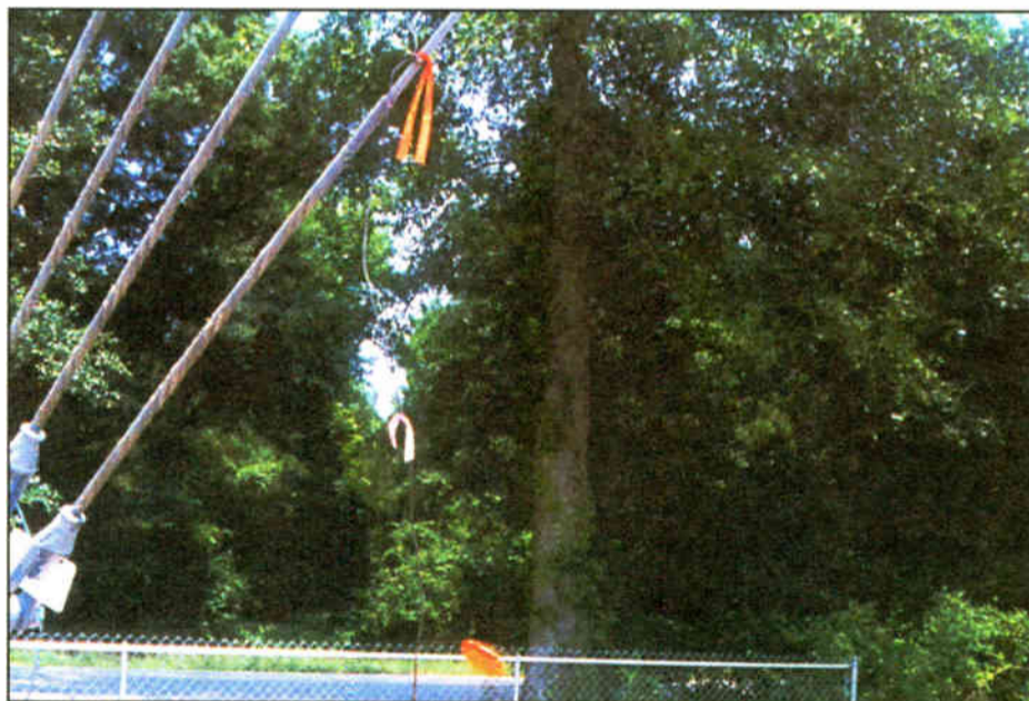
Figure 2: Colored tape marks a ground wire.
