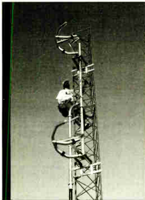
ERI, SHPX series FM Antenna and \lambda Mounting System
