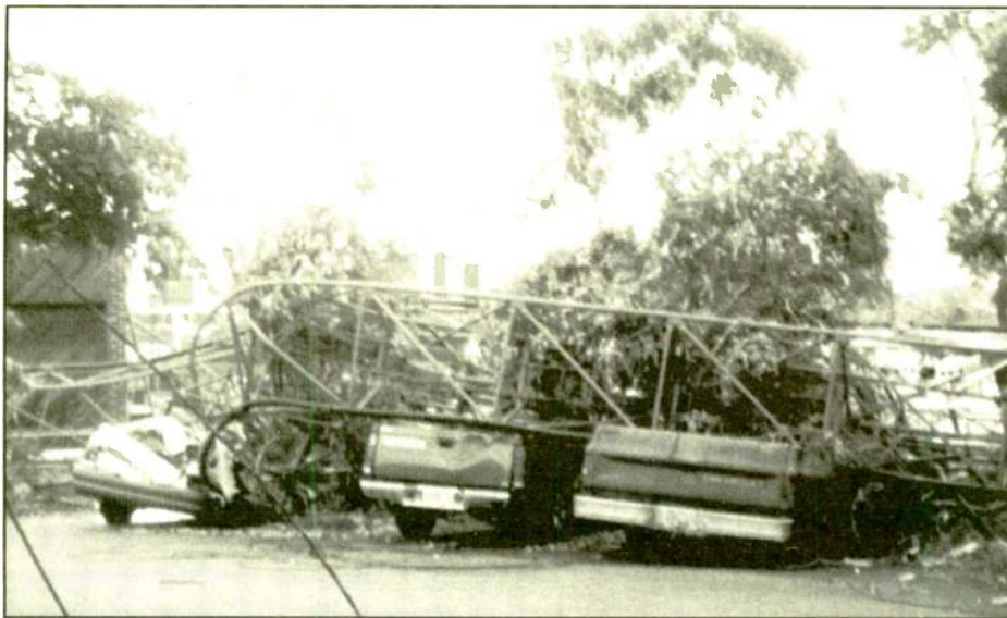
The Chevy pickup drove away from this tower collapse — The new Nissan and the Escort weren't so lucky.
