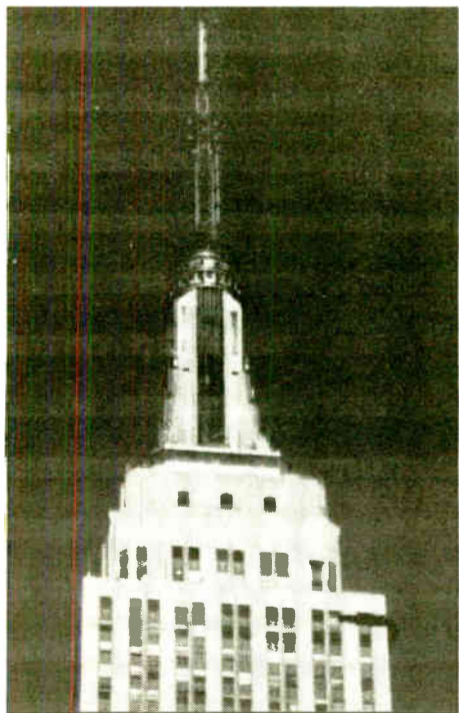
New antenna and combiner system atop the Empire State Building
