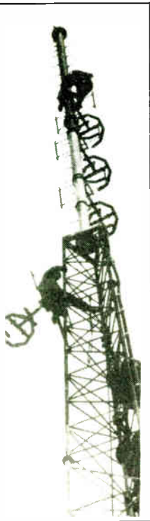
(Above) WAEB's tower: ERI at top; Shively below. (Right) The crew removes the ERI antenna bay-by-bay.
